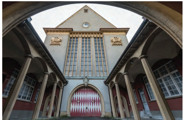
The former Abattoir. Bad Kissingen
